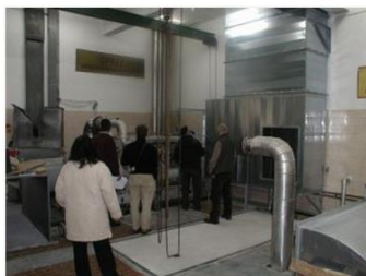
- Gensets for OIV, transmitter stations on top of mountains in Croatia
