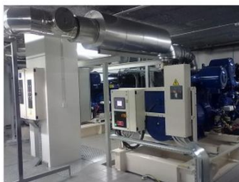
- 6 units 800 kVA prime/900 kVA stand-by with PLC control and Siemens Sivacon S8 TSs for Prompt - Slovenian Telecom main building, Ljubljana, Slovenia
