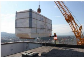
- 6 units 800 kVA prime/900 kVA stand-by with PLC control and Siemens Sivacon S8 TSs for Prompt - Slovenian Telecom main building, Ljubljana, Slovenia
